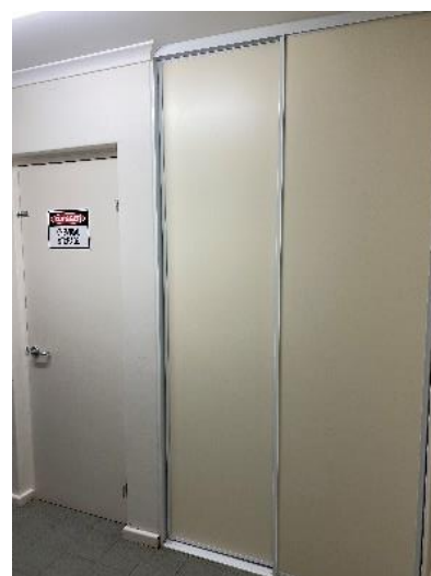
Indoor chemical storage
